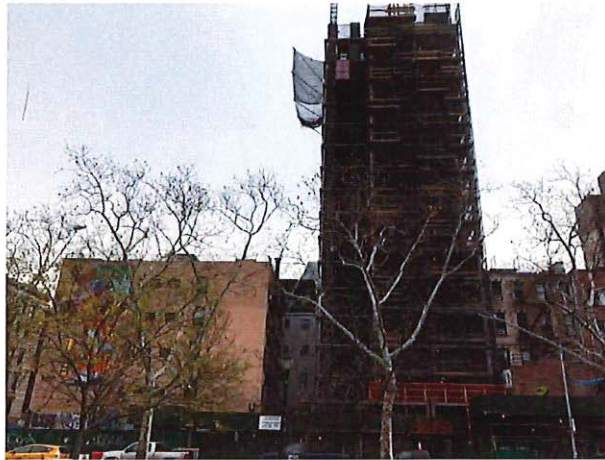
140 Allen Street Main/Hotel Entrance
