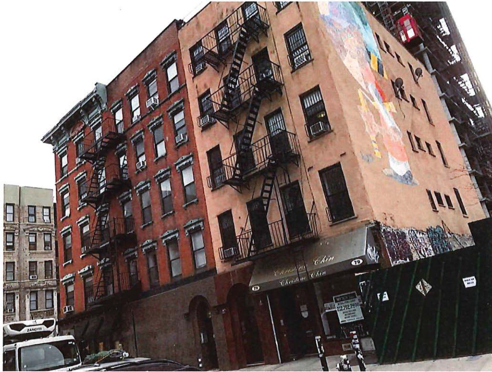
79 Rivington Street Entrance (Space G-2/G-3)
